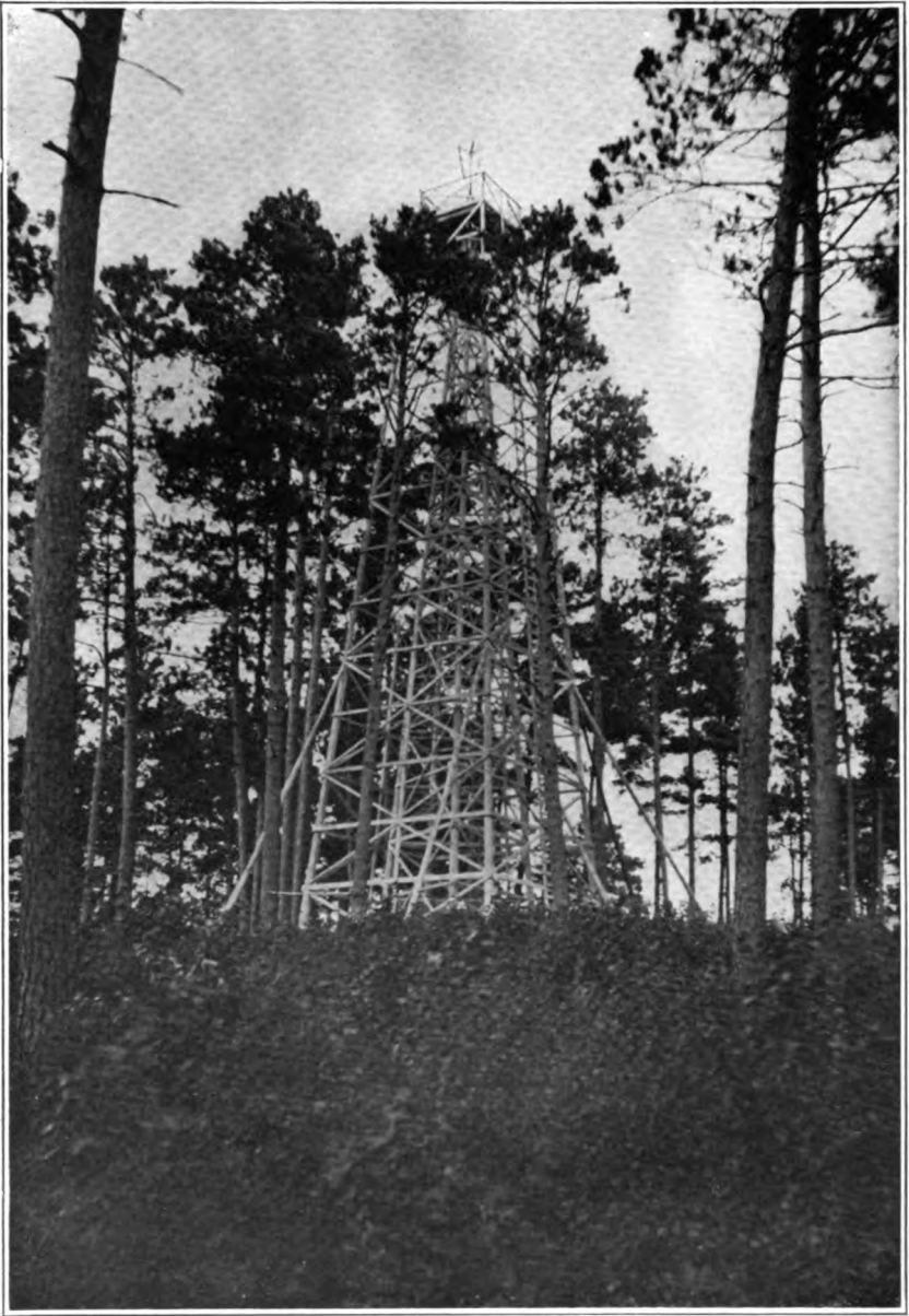
U. S. ENGINEER'S TRIANGULATION PLATFORM AT DEMING LAKE.
